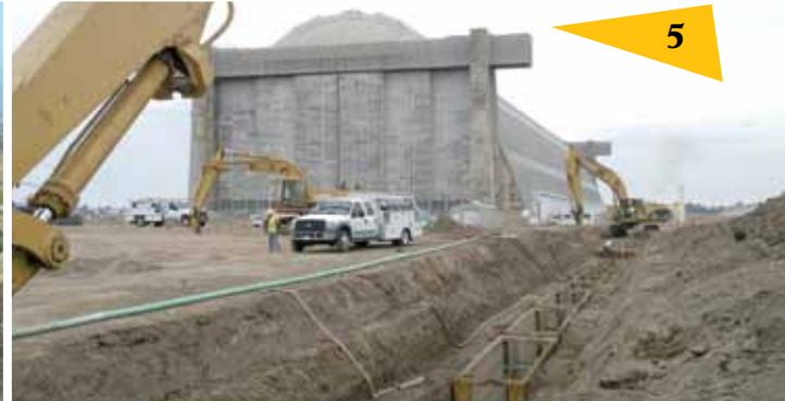
(5) Gwinco installing the sewer line between Tustin Ranch Road & Park Avenue.
